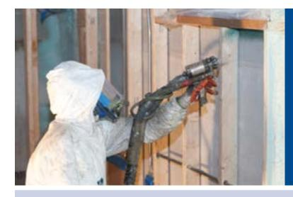
More and more contractors are using spray polyurethane foam (SPF) insulation in residential and commercial buildings to make them energy-efficient. In fact, use of SPF insulation has increased 60% in the last five years. SPF insulates against air, moisture and gas and is often used in perimeter walls, crawl spaces and attics.
